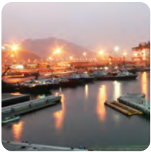
Fujairah Port Expansion
